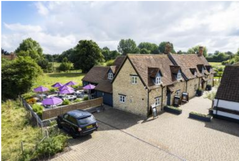
Level Access From Car Park To Entrance
